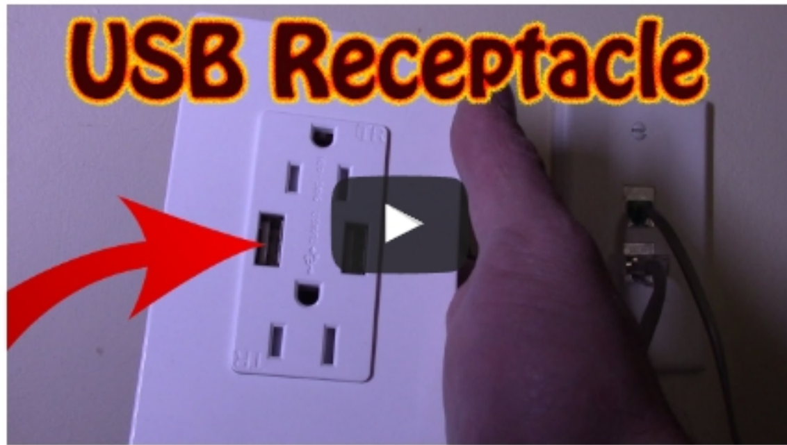
DIY How To Install A High Speed USB Charging Receptacle
